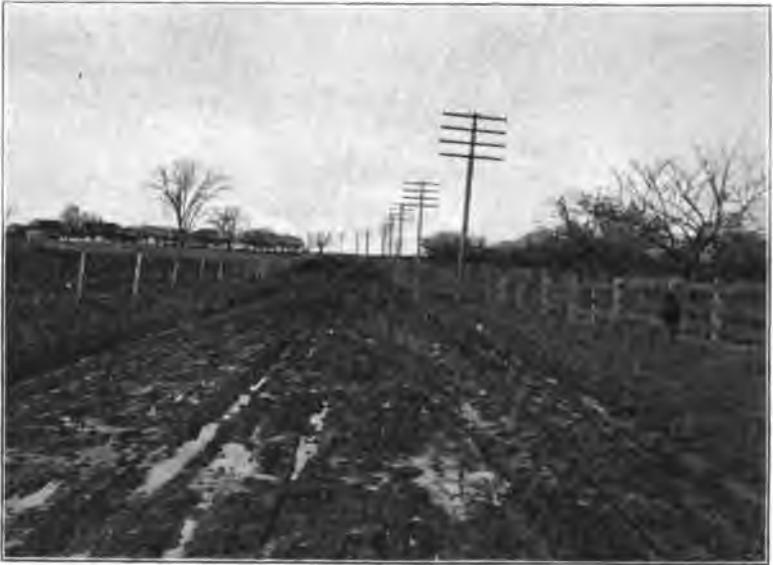
Centreville School House road, Mercer Co., before improvement.
